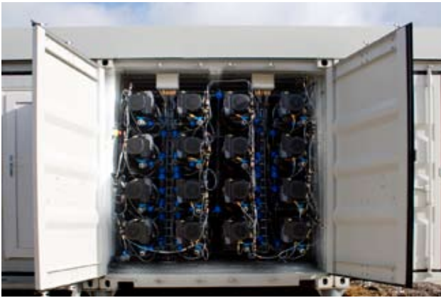
Figure 1 This compact wastewater treatment plant, which can pretreat waste from approximately 1,000 homes, is installed in shipping containers for ease of transport. Photos courtesy of Grundfos
